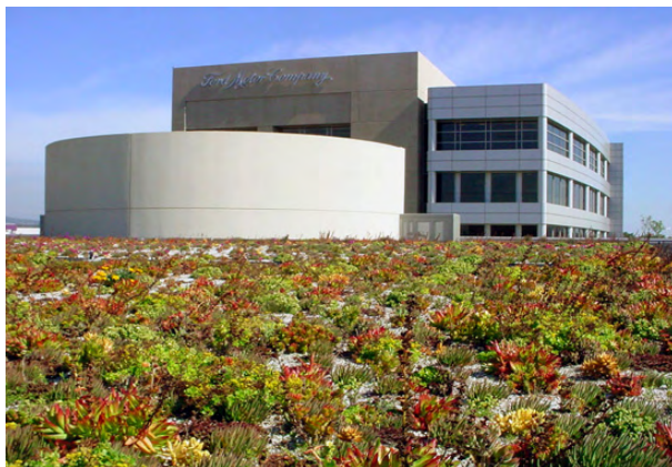
Figure 24: Extensive Green Roof (Sika Sarnafil)
